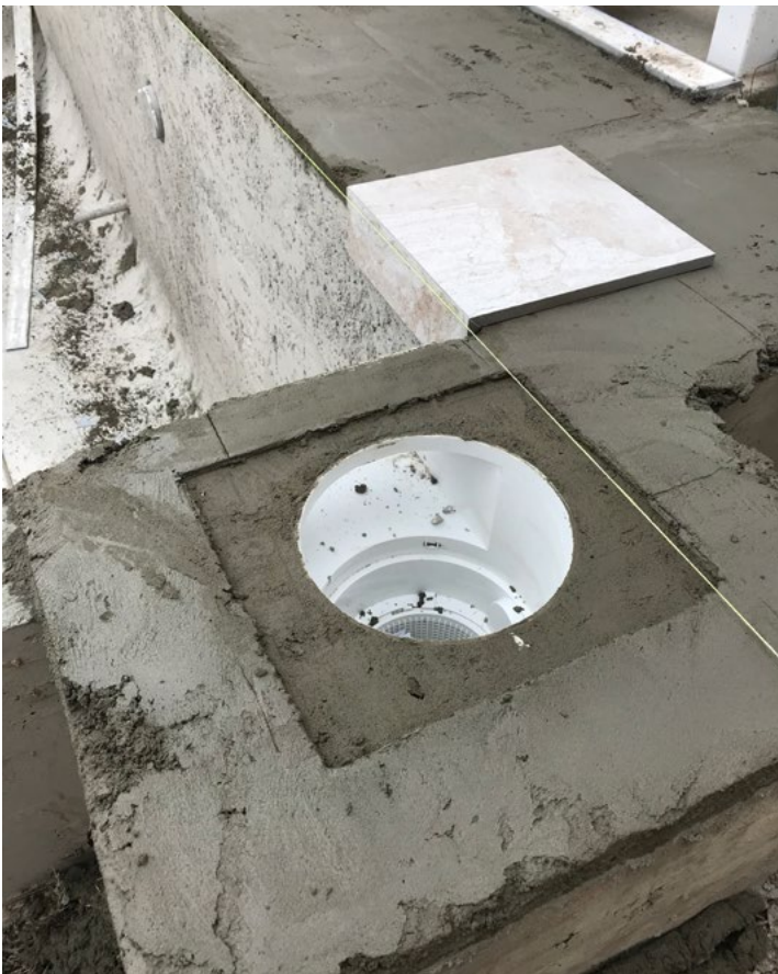
New pool build, allowing for the depth of the Edge Protector
